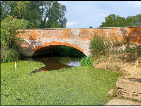
The Hawkeswade Bridge spanning the main stream of the River viewed from downstream across the Hole.
