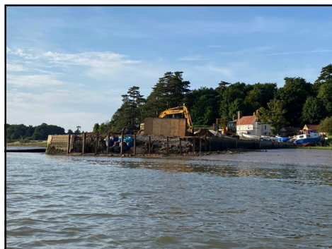
The works at Ramsholt Quay.
