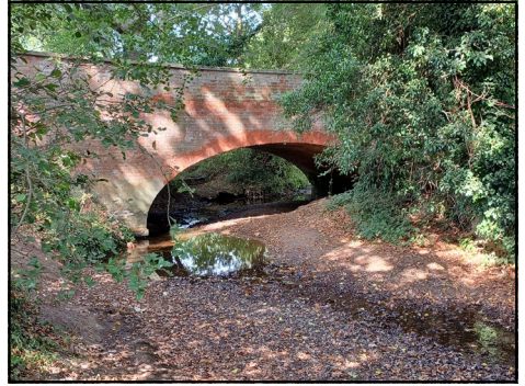
The second arch of the Hawkeswade Bridge spanning the adjacent (nearly dried up) gutterway.
